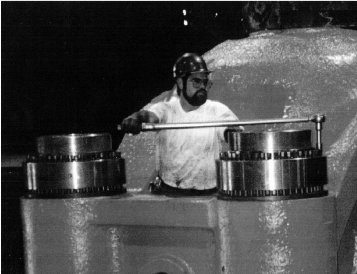
Figure 8. A worker torquing a SUPERBOLT® thrust collar assembly to tension an 18-inch (457.2-mm) tie-rod to a preload of 2,625,000 pounds (11,676 kN). The jackbolt torque being applied with a torque wrench is 275 foot pounds (372.9 NM) SUPERBOLT® Inc.
